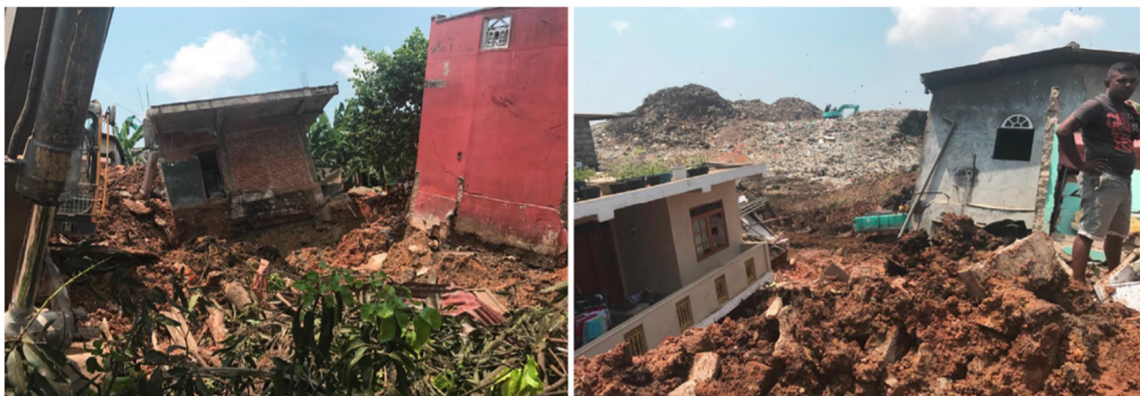
Figure 4. Damage to dwelling units because of the slope failure in Meethotamulla open dump (Jayaweera et al., 2019)
